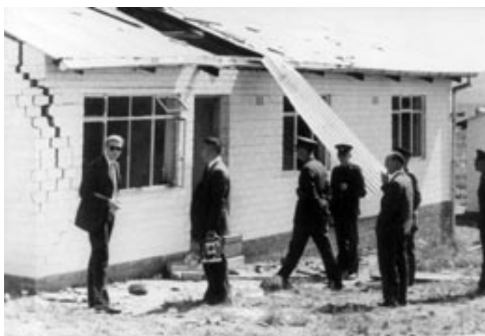
The vandalised house in Laudium
